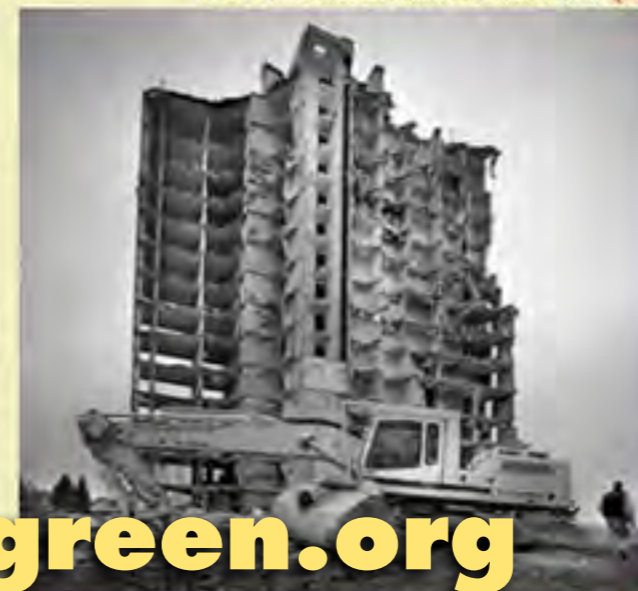
Tours Lavoisier: DURING demolition (F)
