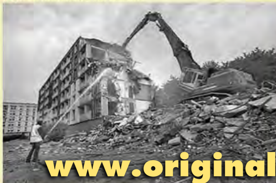
(E) Tours Lavoisier: DURING demolition
