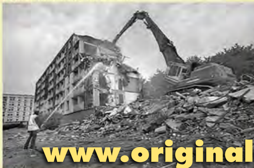
(E) Tours Lavoisier: DURING demolition
