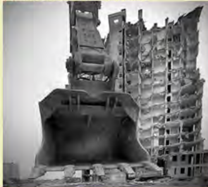
(C) Tours Lavoisier: DURING demolition
