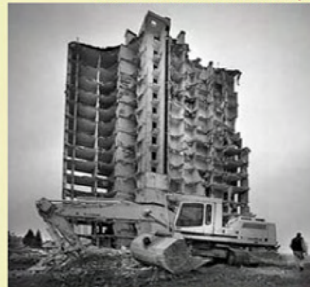
Tours Lavoisier: DURING demolition (F)
