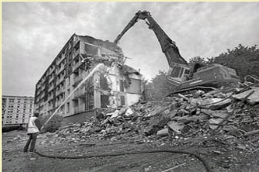
(E) Tours Lavoisier: DURING demolition
