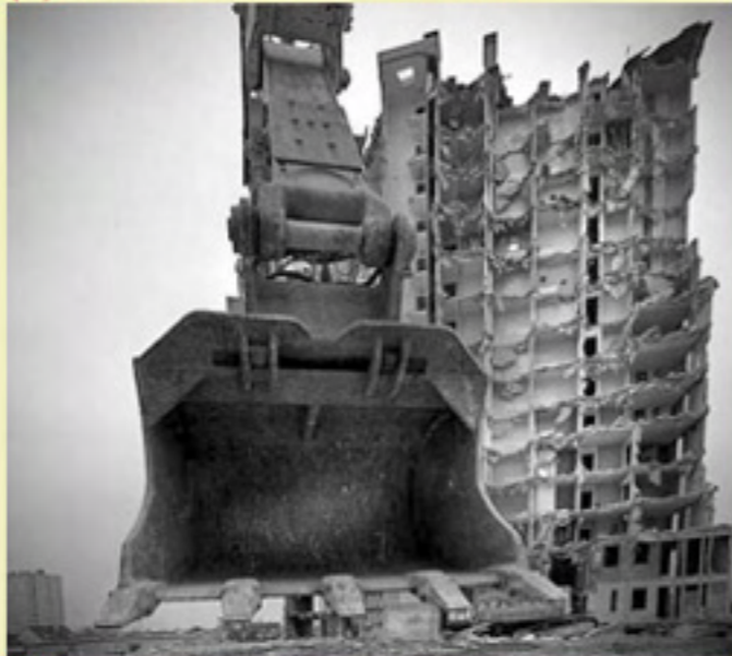
(C) Tours Lavoisier: DURING demolition
